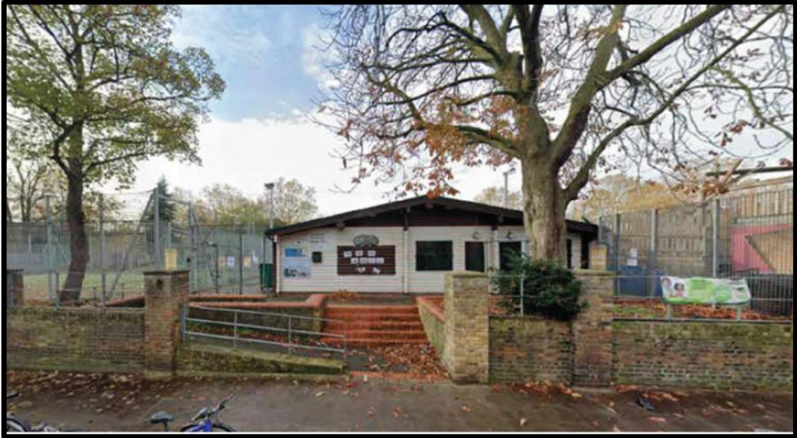
Image 3: Front elevation of existing building.
